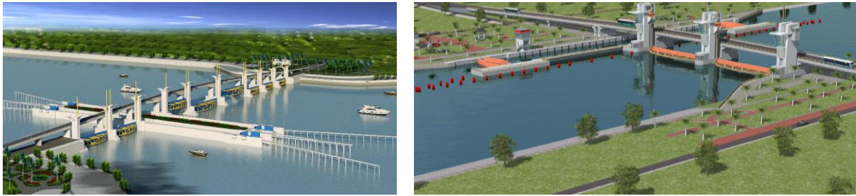
Figure 3. Overall perspective of Cai Lon – Cai Be sluice gates (Source: PMU-10, 2018)
