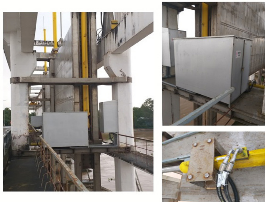
Figure 3-17. Hydraulic cylinders at Lang The sluice in Tra Vinh Province (Taken by the Vietnamese Assessment Team on 23/09/2018)
