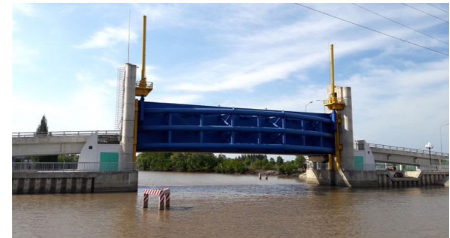
Figure 3-8. The gate of Bao Chau sluice gate (the width of 31.6 m) in Ca Mau
