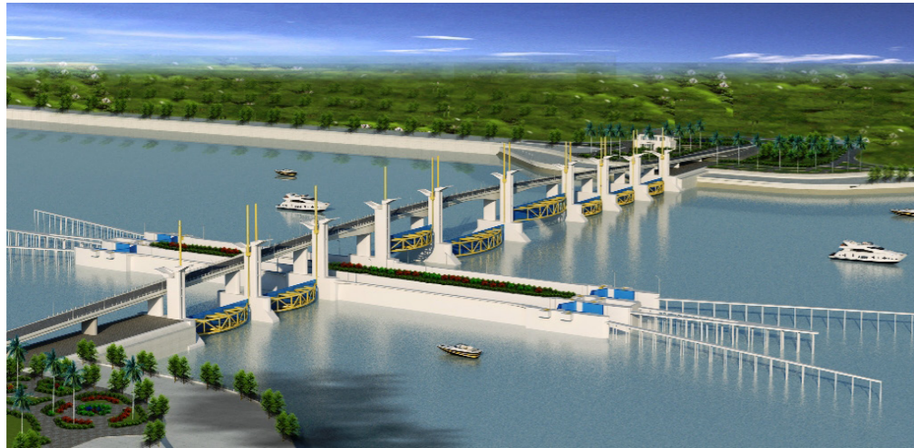
Figure 2-5. Overall perspective of Cai Lon sluice [13]
